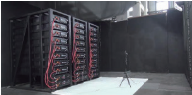
(b) Initiation of venting in Cell 37
