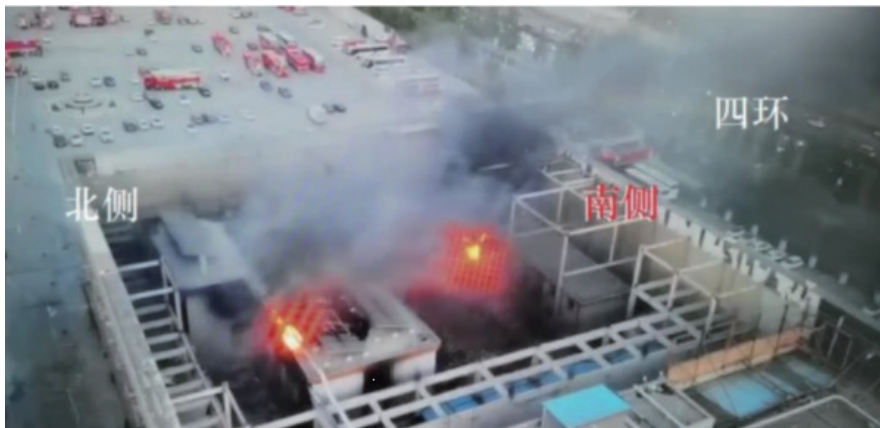
Figure 5 Photograph of the Beijing Dahongmen Accident
