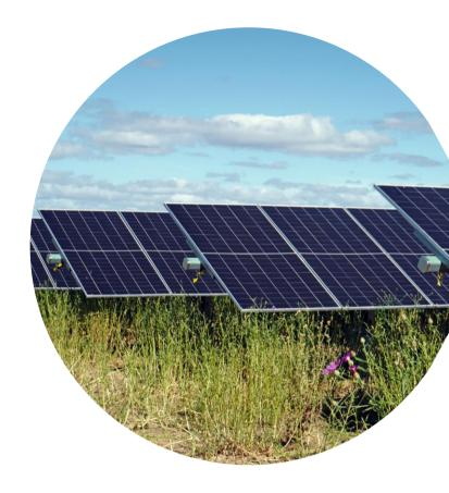
The site at Valcasado is flat and arid, with minimal minor slopes and annual precipitation. These conditions necessitated robust construction, verified by soil saturation and pull-out tests to secure long-term foundation stability. The plant's layout maximizes land use while adhering to legal boundaries, with a tailored mix of 32-module and 64-module trackers to optimize energy capture across three designated zones.
